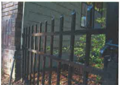
Use non-flammable fencing if attached to the house such as metal.
