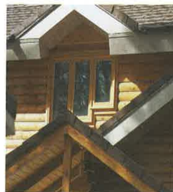
Enclose eaves and soffits.
